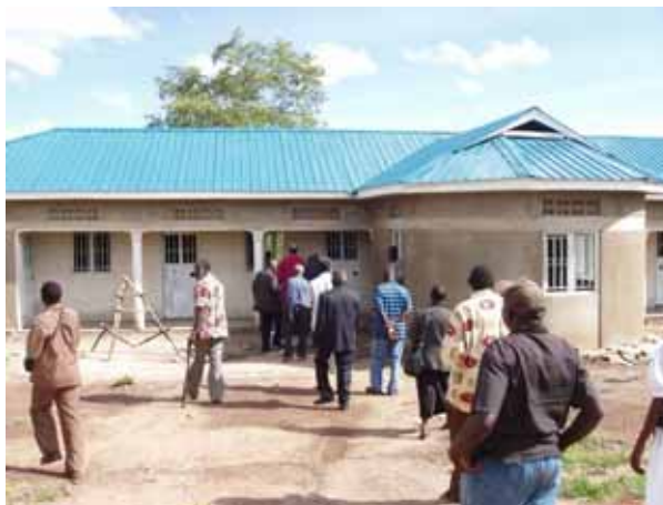
The new Mundri diocesan office building, still in progress.
