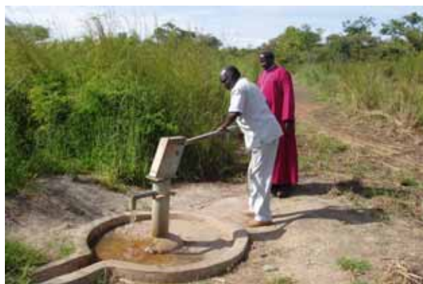
Provincial Secretary Canon Enoch and ++Daniel test the new bore-hole well.
